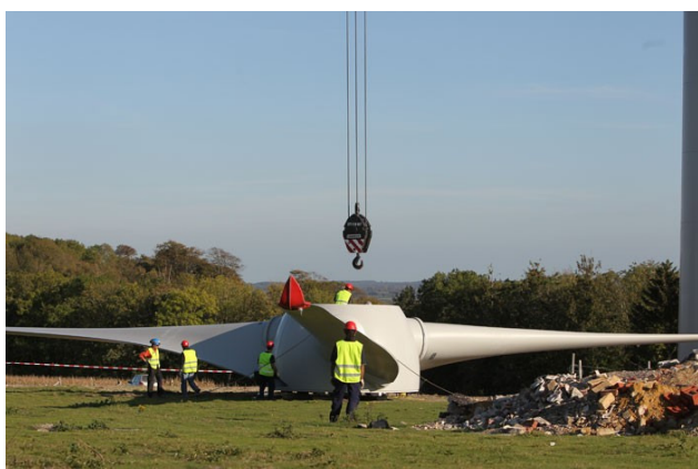
The Glydebourne turbine under construction
